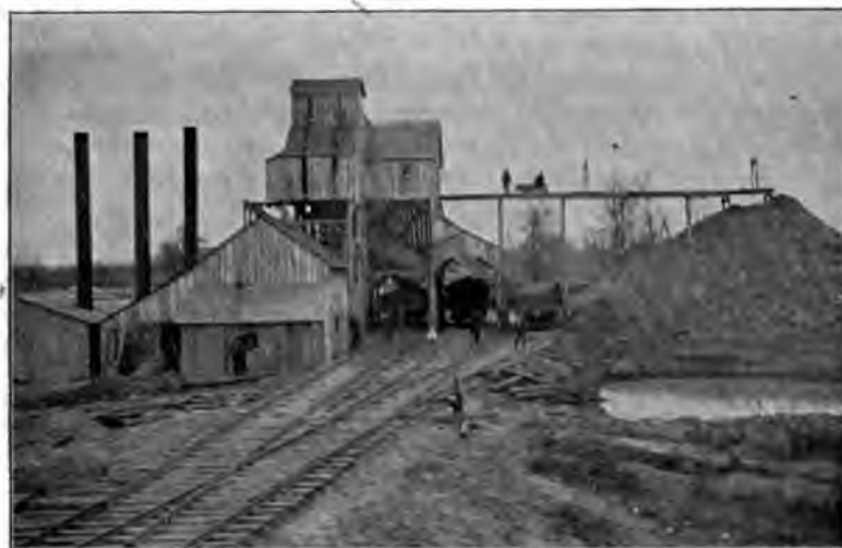
PLANT OF BRIAR BLOCK COAL COMPANY, CLAY CITY, INDIANA.
